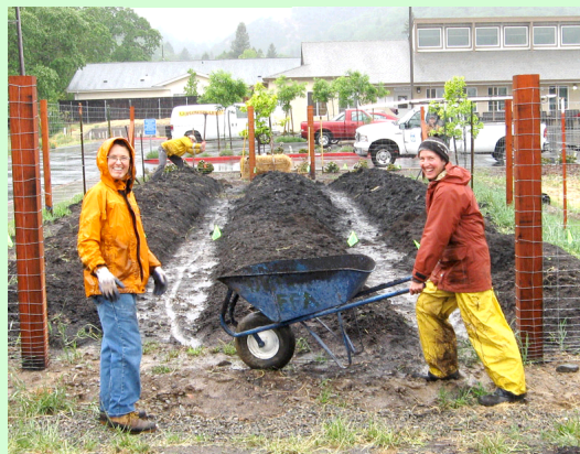
Volunteers successfully created 180 feet of 4-foot wide beds, and also dug trenches for irrigation lines. Photo by Cyril Colonius.
